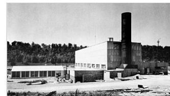
Aircraft Reactor Experiment building at the Oak Ridge National Laboratory (ORNL). It was later retrofitted for the MSRE.
